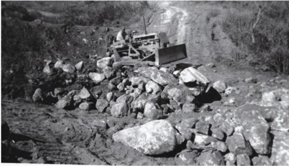
1951 Francis Gillian bulldozing a landing strip for the Waco plane. The 1 st runway was 600 feet along N. Stagecoach Ln. The 2 nd runway was only a 300 foot strip overlooking the Santa Margarita River. (Gillian Collection).
