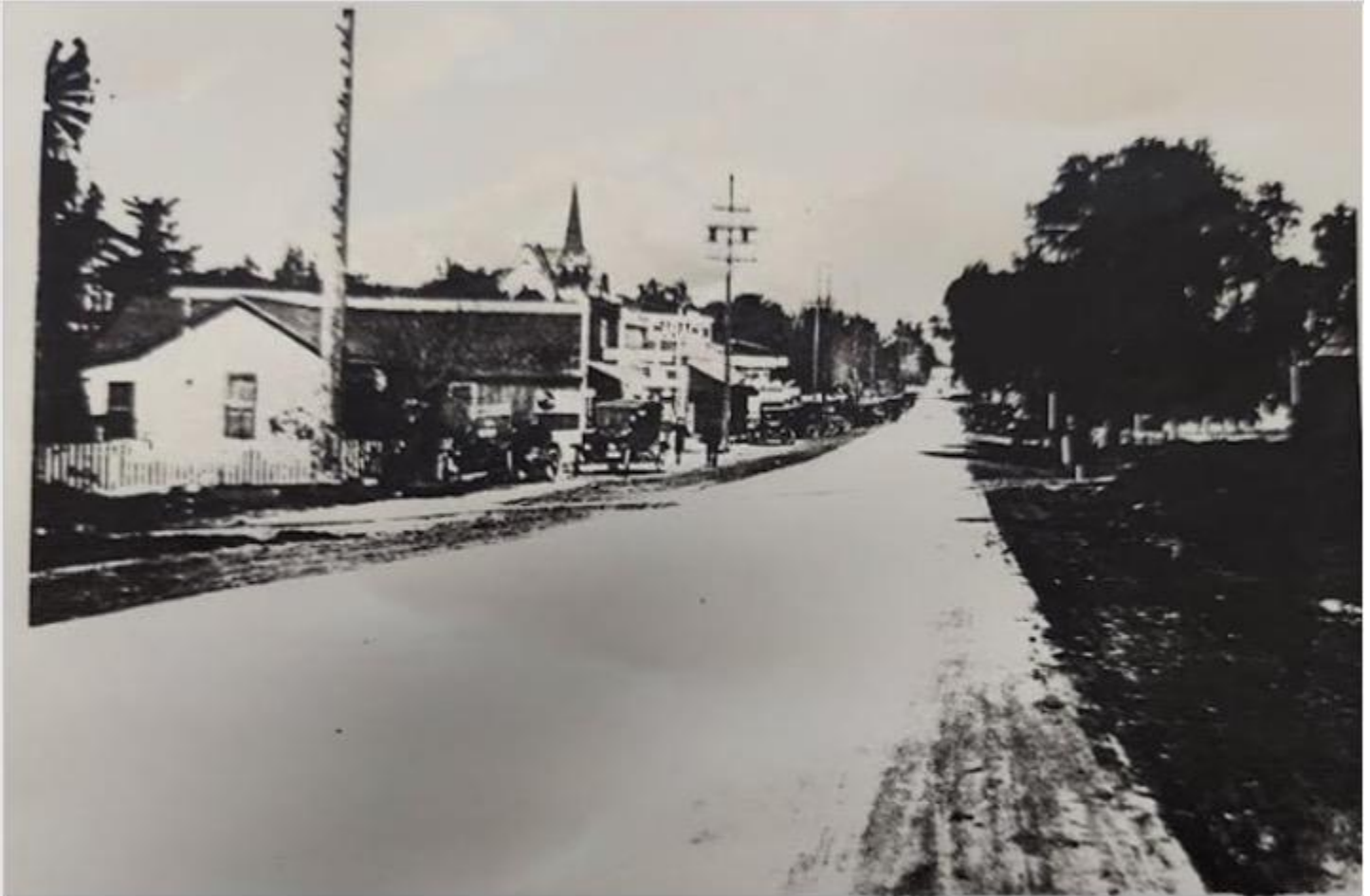
About 1922 Looking north on the Inland highway in Fallbrook at the Main Ave railroad crossing. Two cement lanes are complete. Notice the shade trees along the unpaved dirt parking and pedestrian area along the road shoulder. Fallbrook Historical Society Photo
